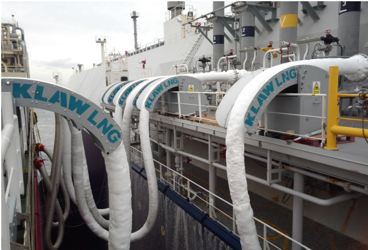
Figure 10 Flexible Hoses during Cargo Operation
