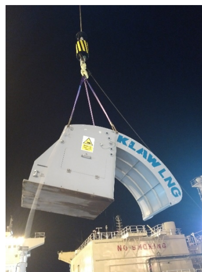
Figure 36 Transfer of Saddles
